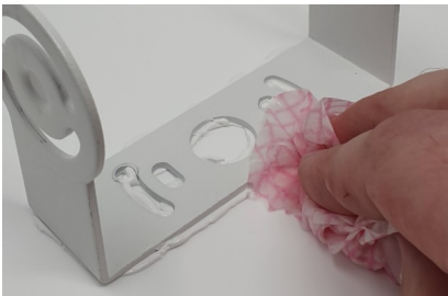
Wipe excess sealant away
